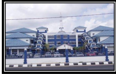
District Police Headquarters for Kota Bharu
